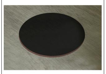
Carve a hole according to the dimension of the LED light on the ceiling.
