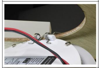
Carefully place the LED driver through the hole and securely hook the spring frames onto the edge of the carved hole.
